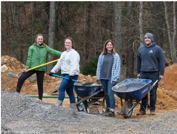
Campus Ministries at Grand Valley State University sent the only mission team to CMMBC in early March of 2020. Students are shown here as they helped to get ready for pouring concrete for the splash pad.
